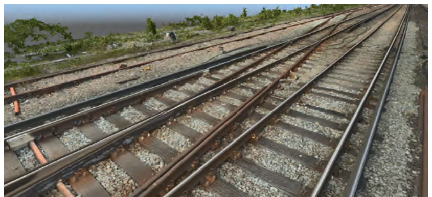
▲ Unlike with traditional methods of conducting railway surveys, topographical survey CAD data is complemented by ultra-high-resolution orthophotos and highly detailed coloured point clouds as well as the RAW photography.
